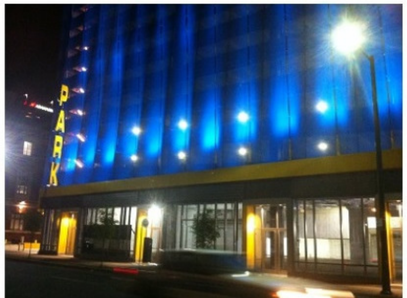
*ACTUAL PICTURE OF PARKING GARAGE*
