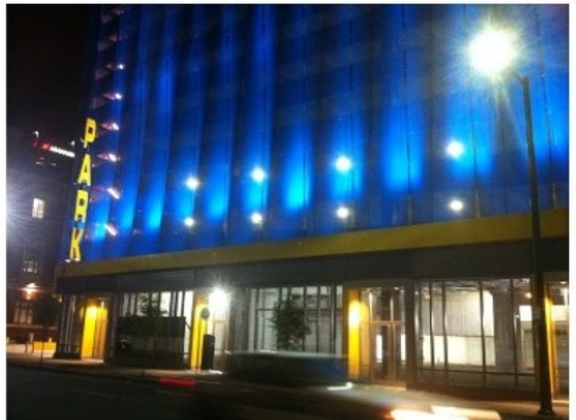
*ACTUAL PICTURE OF PARKING GARAGE*
