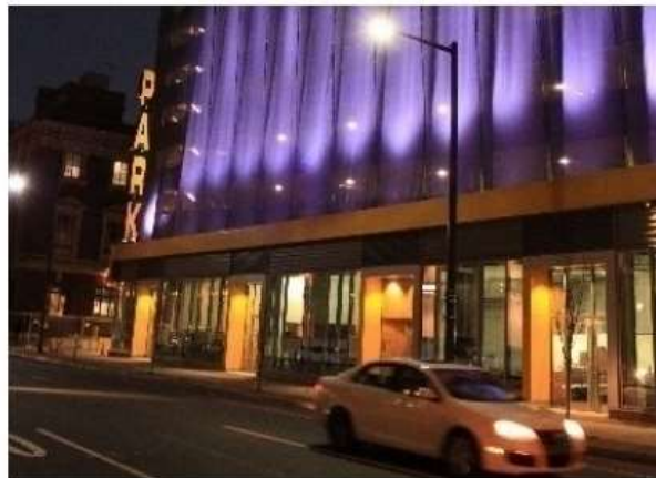
*ACTUAL PICTURE OF PARKING GARAGE*
